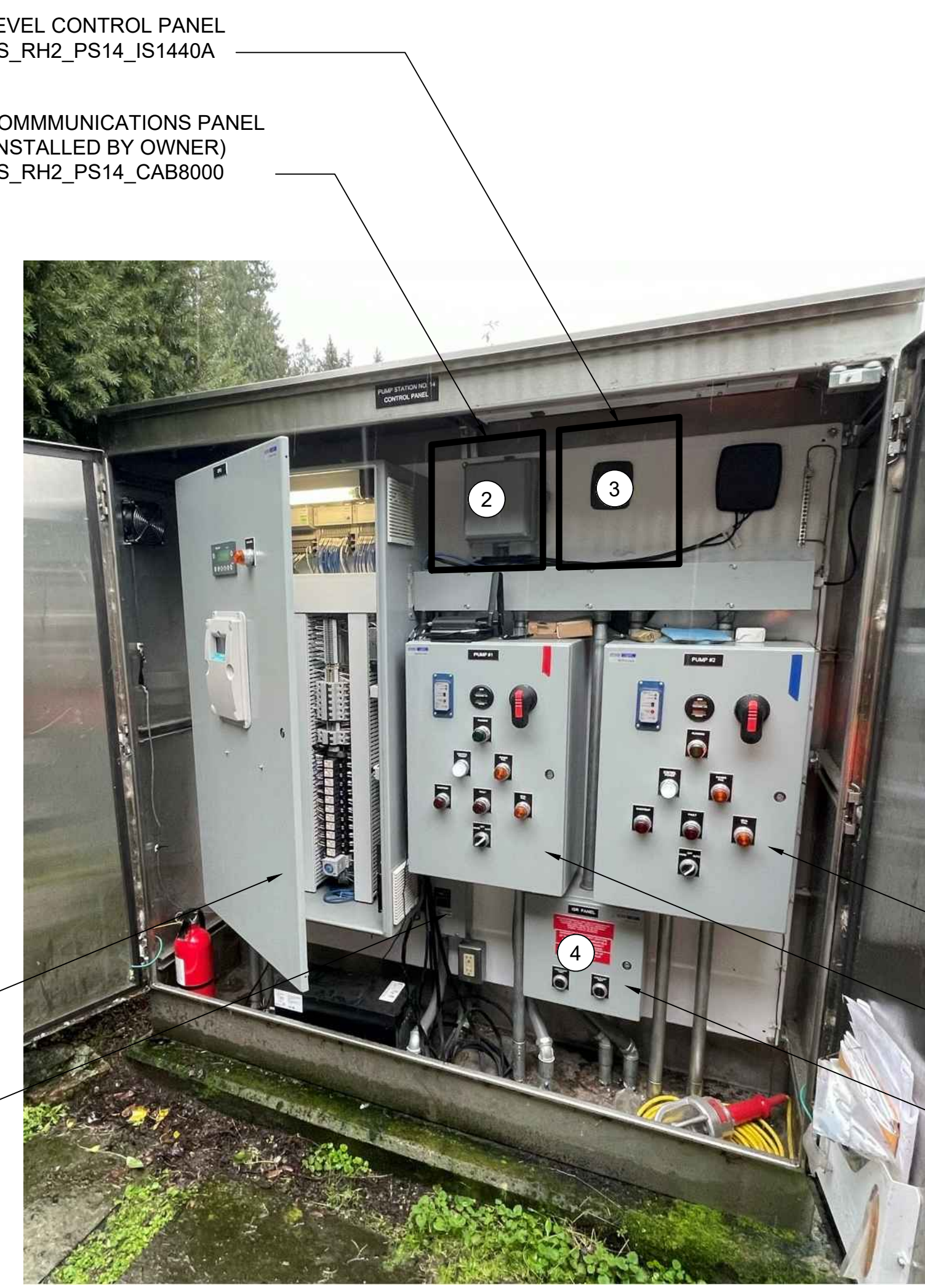
PUMP STATION CONTROL PANEL LAYOUT
